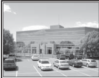
104 Interchange Plaza, Cranbury 4,160 SF & 12,419 SF
