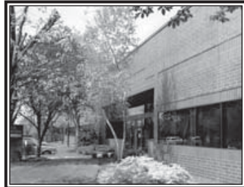
North Brunswick Commerce Center 100 North Center Drive, North Brunswick 2,472 SF, 5,007 SF & 8,589 SF
